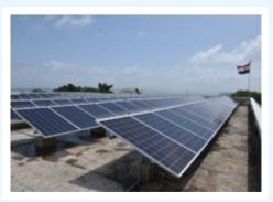
The two rooftop grid Solar Power Plants are set up at the Port Administrative building and the other at the Port Hospital building, covering an area of 4300 square metres, both having a combined capacity of generating 1000 kwh/day approximately.
